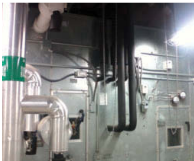
Refrigerant piping penetrating the AHU upstream of the pre-cooling coil.
