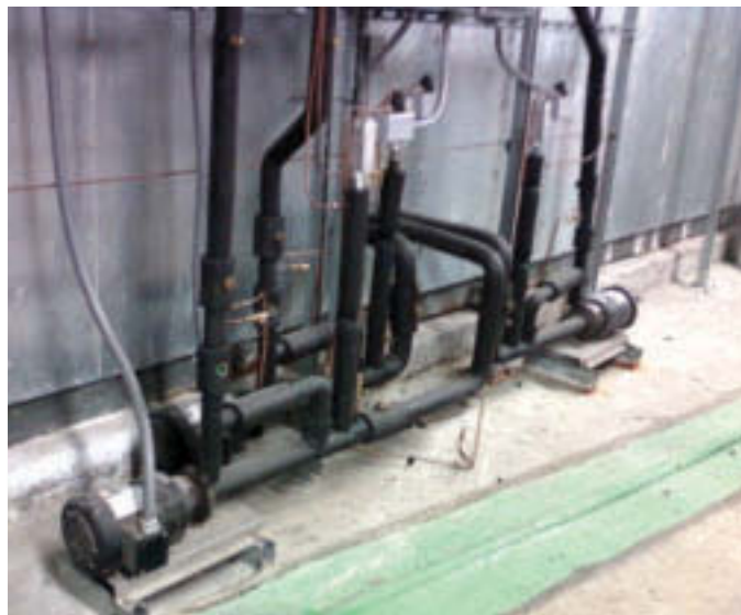
Pumps that assist in moving the liquid refrigerant up to the upper coil.
