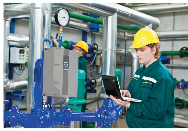
A recent development in hydronic systems has been the emergence of "sensorless" pump control, offered by several manufacturers. Sensorless pump control typically consists of a pump packaged with a pump-mounted VFD (Variable Speed Drive), supplied and programmed by the manufacturer, offering variable-speed control of the pump without the need of a downstream differential pressure transducer.
